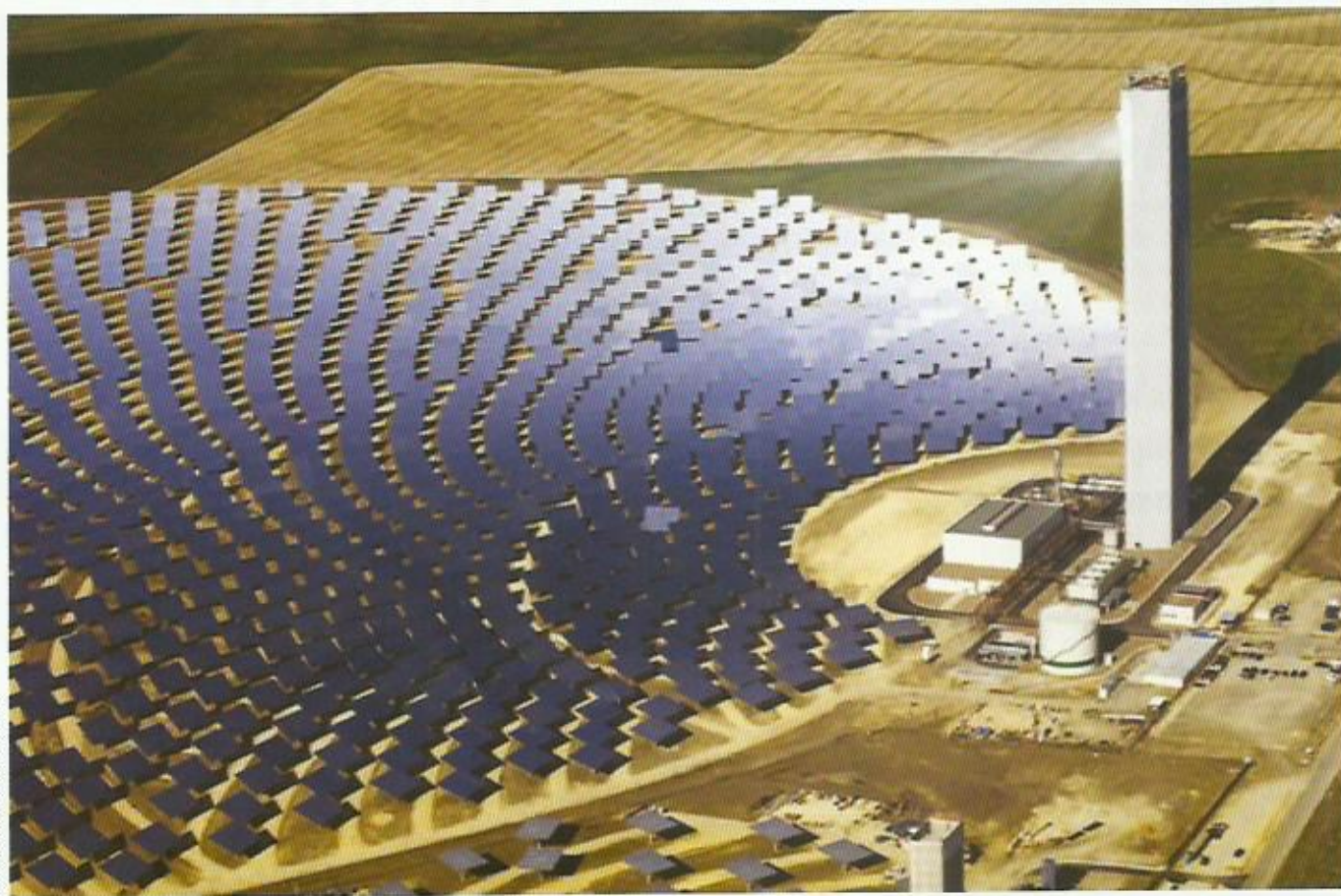
A sea of mirrors directs a powerful beam of light toward a solar power tower...
