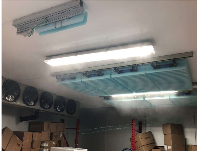
Figure 2: Actual representation of TES system in a warehouse.
